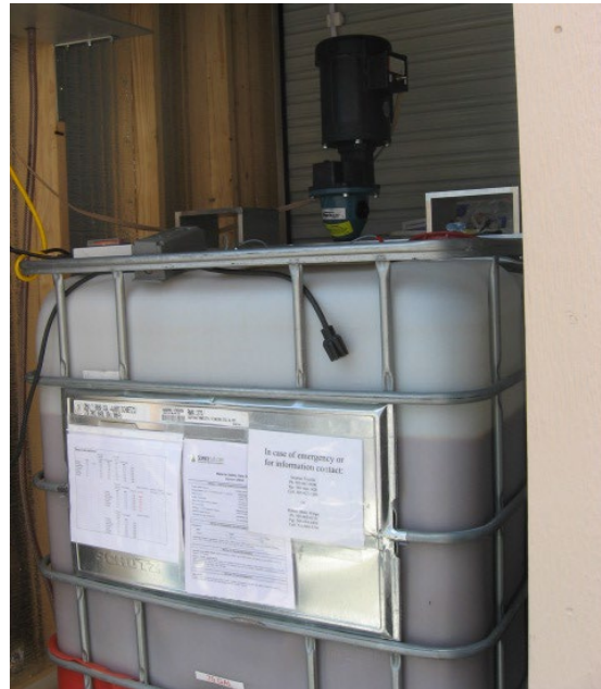
Photograph - NPDES-13S-18-009 SWWS Glycerin Feed System
