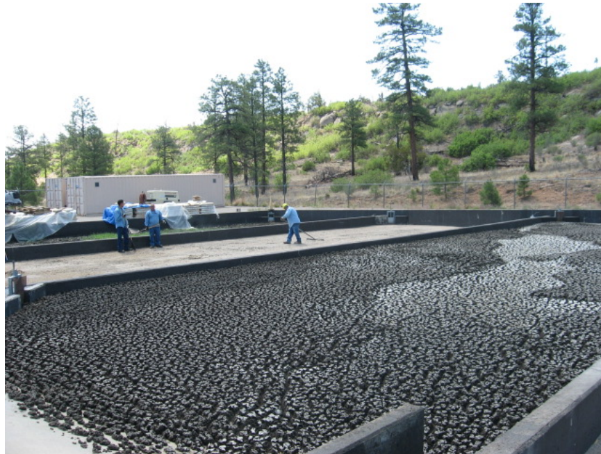
Photograph - NPDES-13S-18-020 SWWS Sludge Drying Beds
