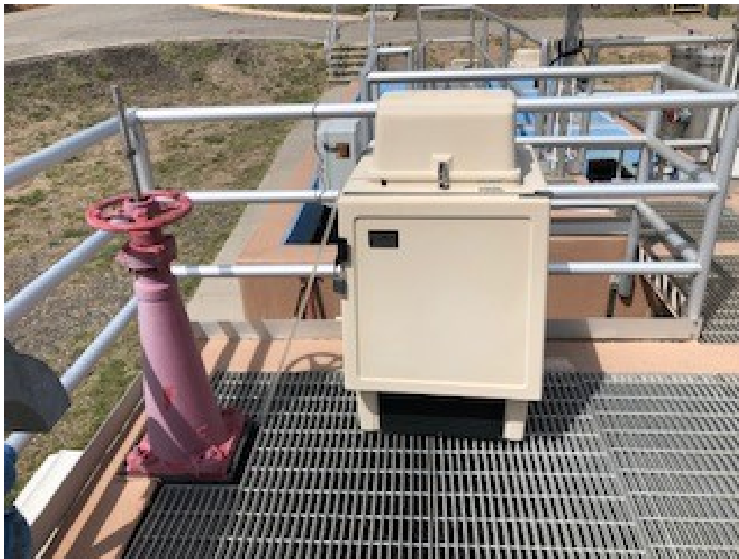
Photograph - NPDES-13S-18-004 Outfall 13S Ability to Collect Representative Operational Samples at the Chlorine Contact Chamber
