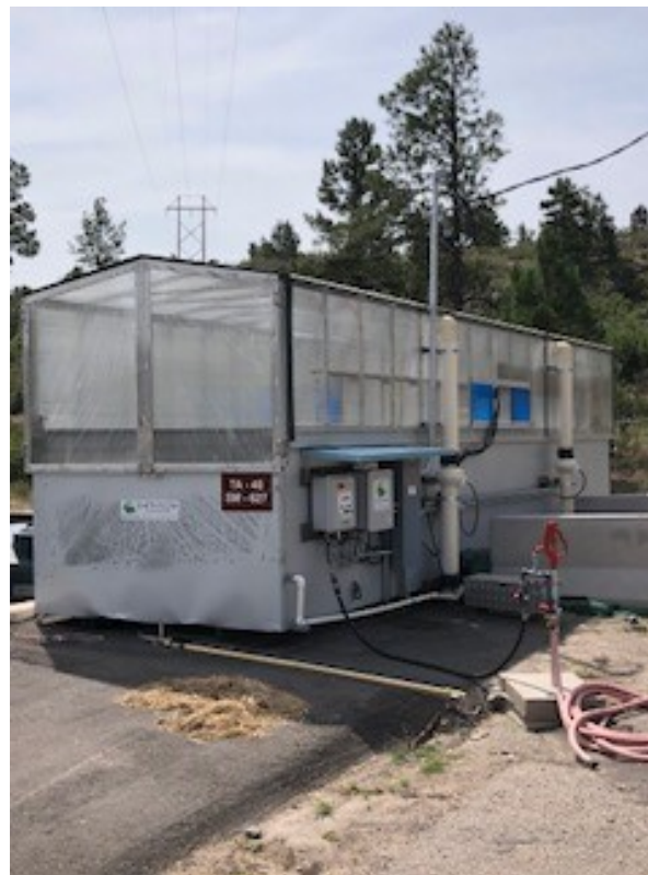
Photograph - NPDES-13S-18-021 SWWS Sludge Composting Structure
