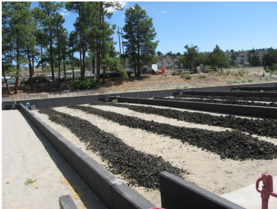
Photographs - NPDES-13S-18-019 SWWS Sludge Drying Bed Winrow Composting
